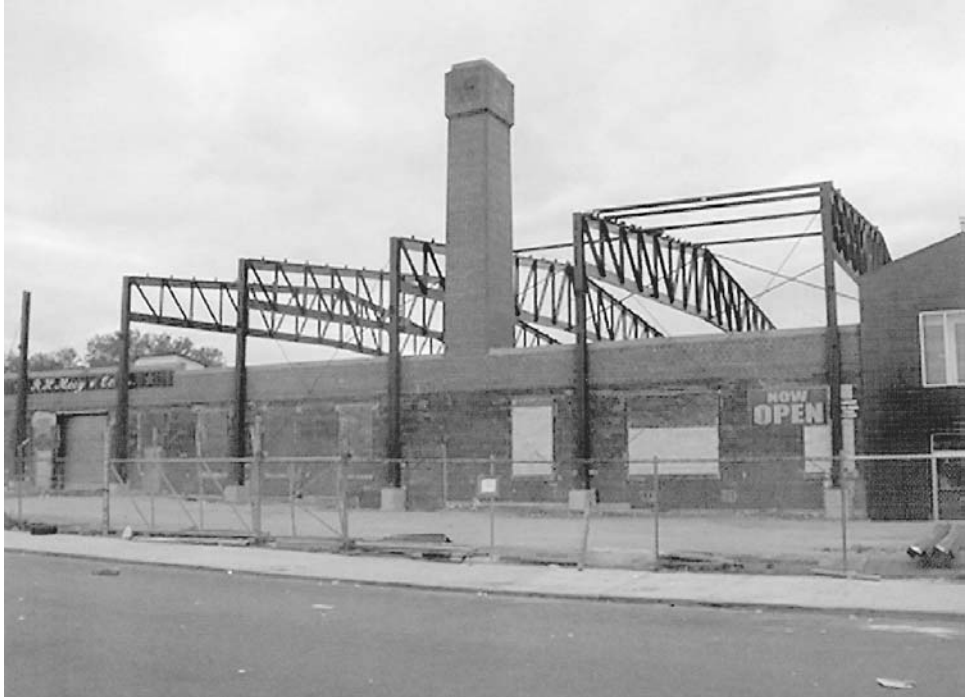
FIGURE 14.13 Proprietary framing envelops an old building. ( Coronis Building Systems .)
