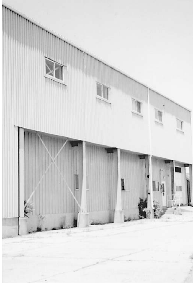
FIGURE 14.12 Second-story addition above existing metal building.
